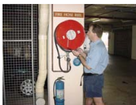
Maintaining a hose reel to AS1851
